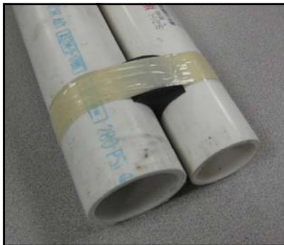
3. Secure the SPACER PLUG in place with a few wraps of heavy tape. This aligns the pipes and prevents them from spreading during backfill.
