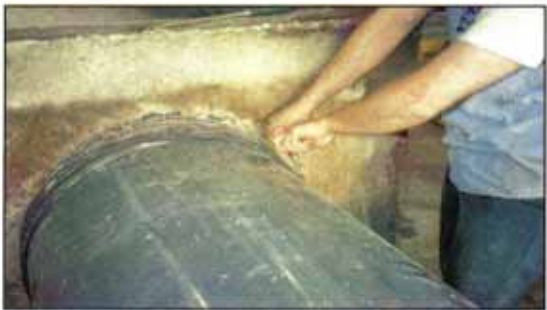
Field Installation: Tighten down take-up clamps with a T-Torque Ratchet set to 60 lb/in. Screw housings should be opposite each other, or on the quadrants, to equalize installation pressure.
