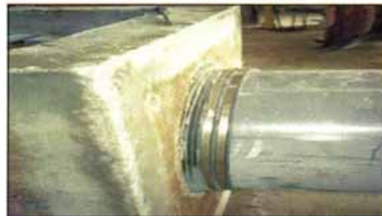
Now you're ready with a flexible, watertight connector.
