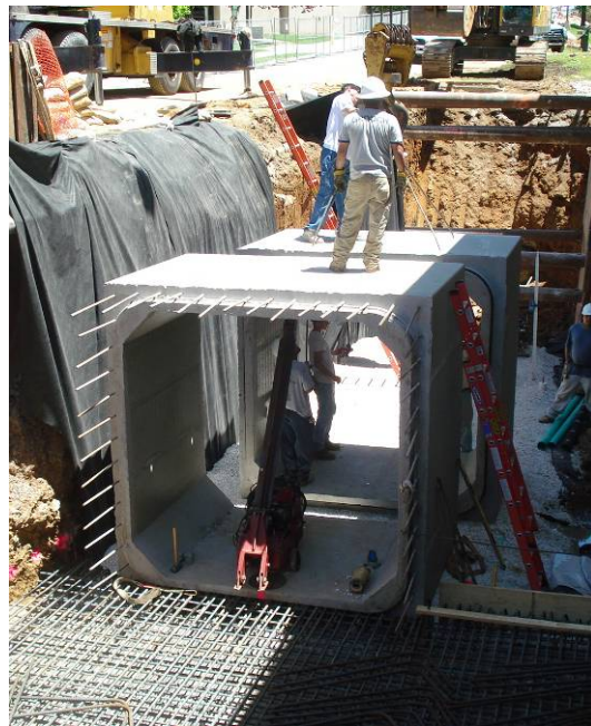
Joining the First Gasketed Joint
