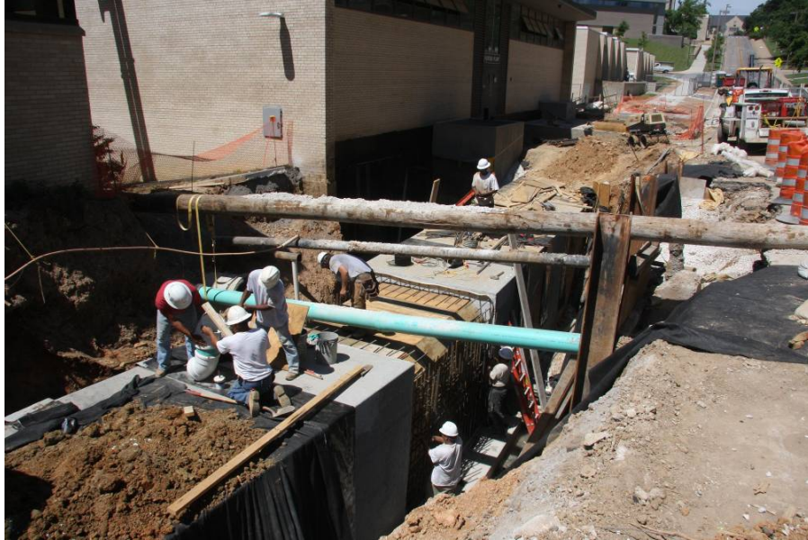
Dodging Existing Utilities in Narrow Work Area
