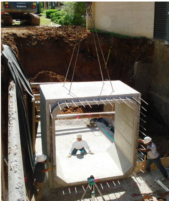
Setting the First Section
