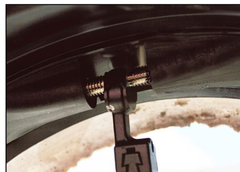
**5. Begin to tighten the Nylo Drive™ Connector by pulling the wrench handle toward the outside of the manhole. The wrench will ratchet back easily at the end of the stroke.**
