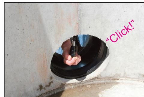
*To remove an installed Nylo Drive™ Connector, simply reverse wrench position and loosen Connector. Connector may be reused without further adjustment.*
