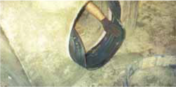
STEP 8: Unfold the CAST-A-SEAL
