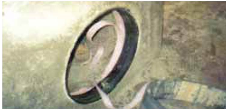
STEP 7: Remove foam material.
