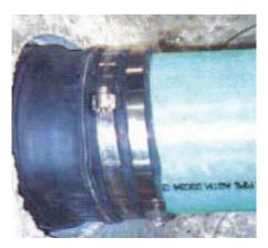
Contractor: To install pipe, align pipe carefully with Connector opening and push pipe through until inside plane of manhole wall is broken as required. Support pipe in center of Connector and attach take-up clamp(s) to connector clamp grooves. Tighten each take up clamp to 60lbs/in torque, using a torque-limiting ratchet or other suitable method. Backfill and compact soil as required
