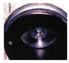
Place assembly in form at proper position and orientation and secure to form using magnet, wire or other secure method. Pour concrete and vibrate adequately completely around key-lock area of Connector to consolidation of concrete all around the Connector.
