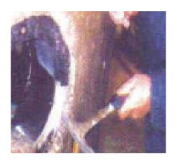
Remove Mandrel to outside of manhole.
