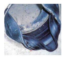
Unfold (flip) Connector toward manhole outside. Remove any debris that may be on or in Connector. Connector is now ready for pipe installation.
