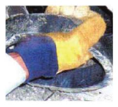
After manhole is cured for stripping, remove form(s) and pull casting ring free from the assembly toward inside of manhole.
