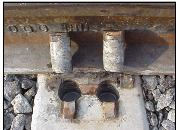
Broken double shoulder cored out of a concrete tie in 1 minute using Corefast diamond core drills on a double head drilling machine
