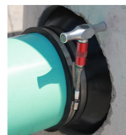
Expansion mechanism at bottom is for display purposes only. Press-Seal recommends installation between a 10:00 and 2:00 position.
